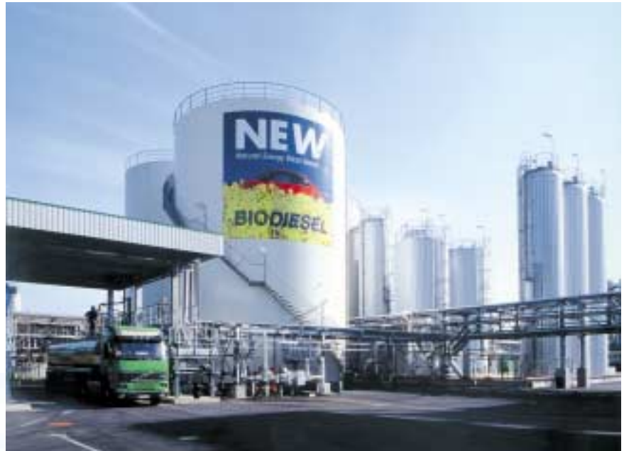
Biodiesel plant Marl, Germany Capacity: 100,000 t/y
