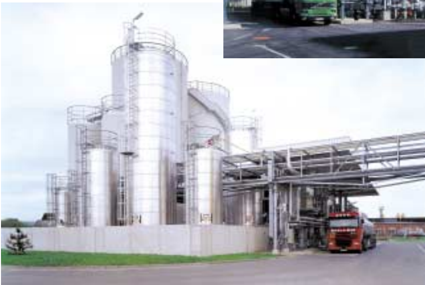
Biodiesel plant Malchin, Germany Capacity: 50,000 t/y
